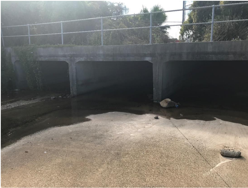
Figure 2.2. Existing Box Culverts
